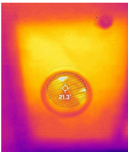
Thermal Image 1 The fan needs a non-return fan cover and the insulation replaced (the yellow should be purple)
